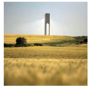
image View across a field of the 115 metre (377 foot) high tower at the PS10 Concentrating Solar Power Plant, in Seville, Spain. Below this tower 624 large movable mirrors called heliostats concentrate the sun's rays to the top of the tower where a solar receiver and a steam turbine are located. The turbine drives a generator, producing electricity. (C) Greenpeace / Markel Redondo
